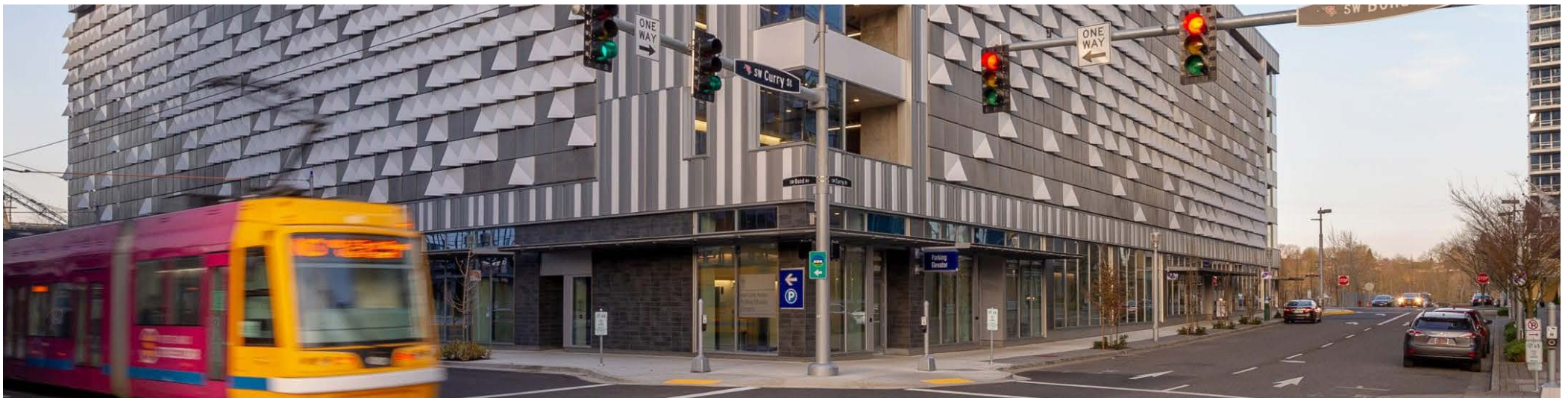
Gary and Christine Rood Family Pavilion - Portland (ZGF Architects)
