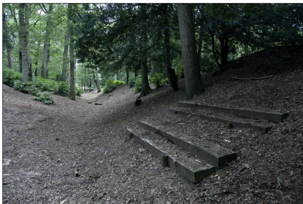
25.2 Channel up to 3 m deep excavated to allow the water to cross a low hill at the Mariënboom component part (25a).
