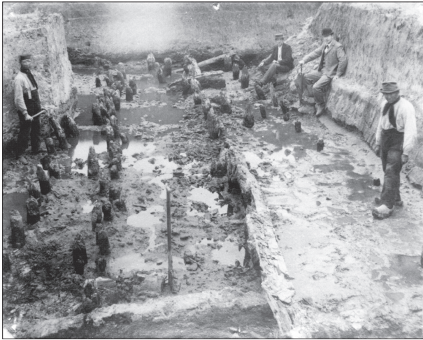
16.3 View of an excavation in 1892. Timber posts and revetments protecting the bank of the Roman Rhine. Seen from the west
