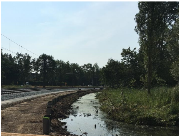
Nieuwe damwand in IJsselstein (tracé D)
